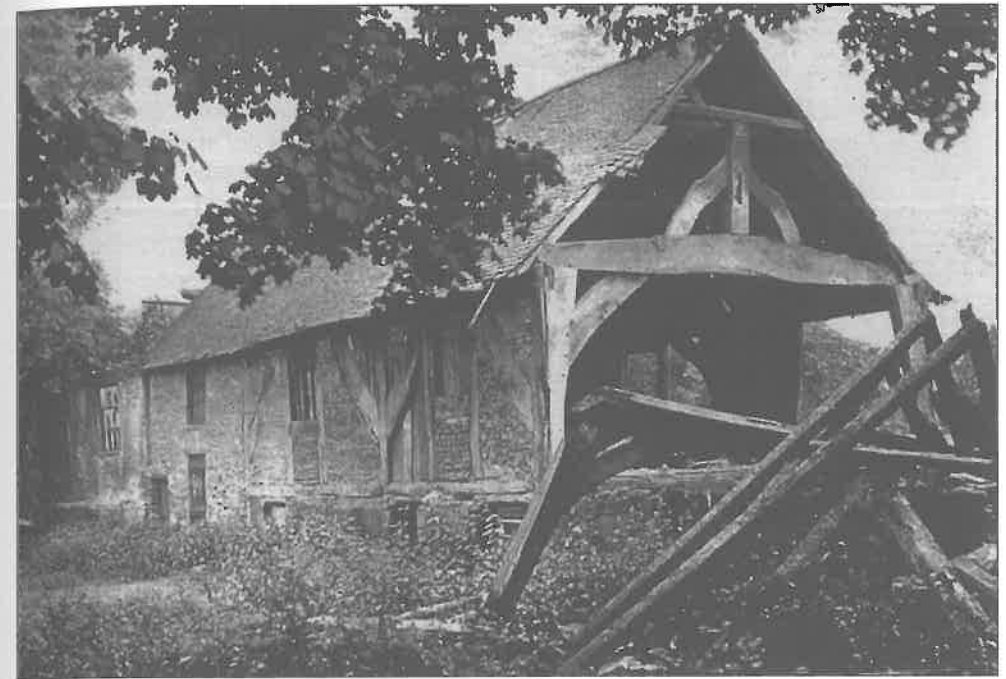
32. Guest accommodation at Basingwerk Abbey.
