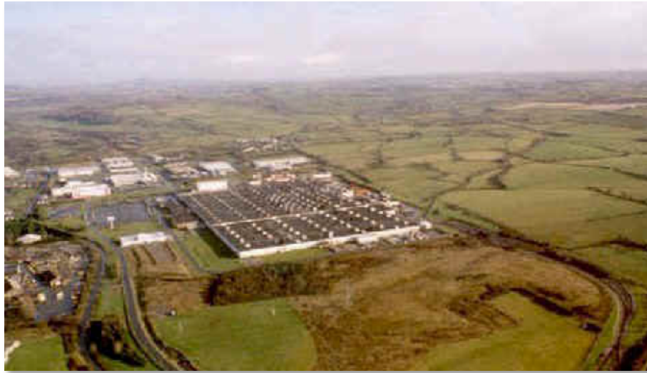
Figure 1.5 - Bridgend Engine Plant (Ford Motor Company, 2017)
