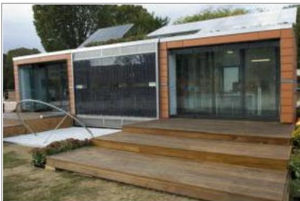
Photo: Passive solar gain: the large glass windows in this spacious wooden building help to absorb heat energy from the Sun. Picture by Donald Aitken courtesy of US Department of Energy/National Renewable Energy Laboratory (DOE/NREL) .
