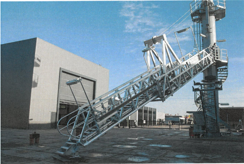
Figure 3. Gangway Solutions who supplied Dragon LNG it's Gangway. ✓
