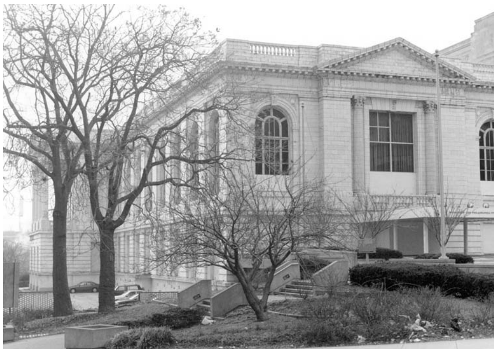
Figure 31. The sad state of the Commercial Museum, shortly before demolition. Photo: Steven Conn.
