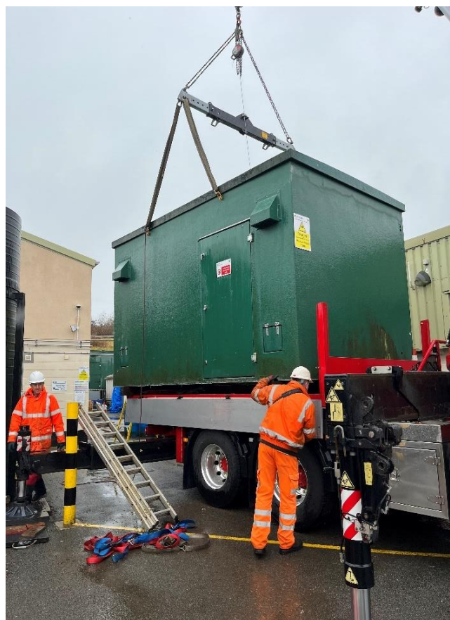
Figure 33 Jekko SPX532 placing the enclosure on a flatbed trailer
