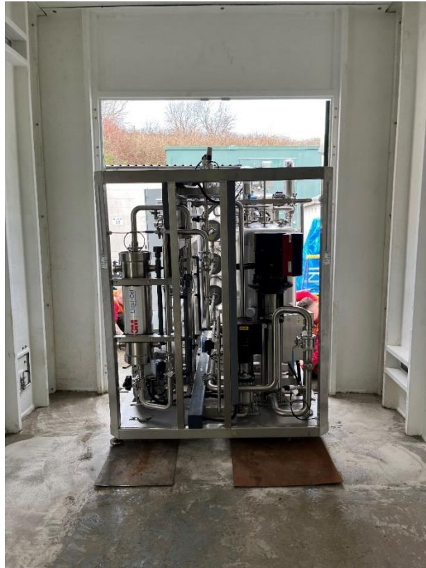
Figure 40 Orion being positioned in the new enclosure
