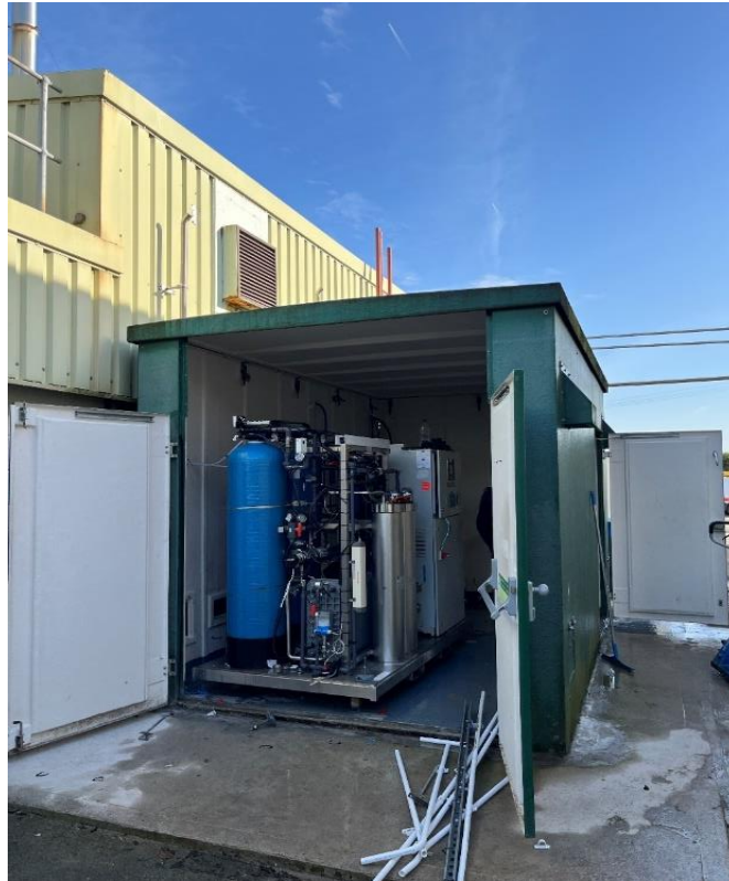
Figure 28 The removal of the Quattro from the glass reinforced plastic enclosure.
