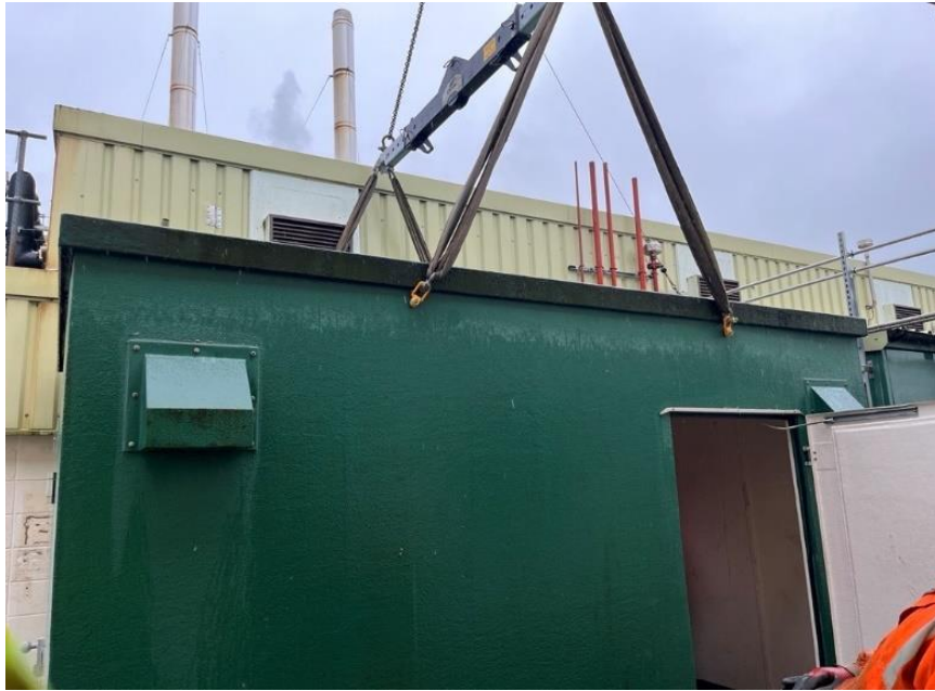
Figure 31 Jekko SPX532 preparing to lift the enclosure
