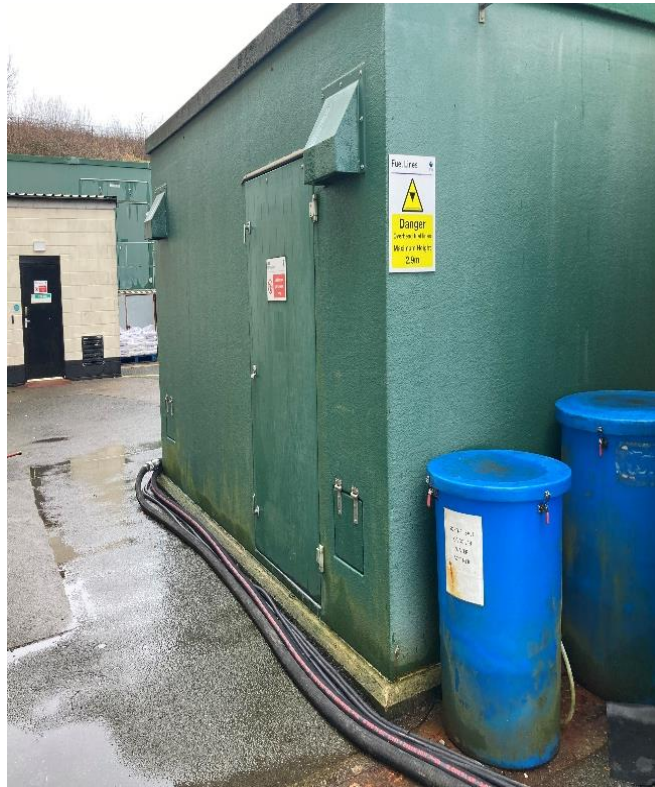
Figure 22 Existing enclosure side view
