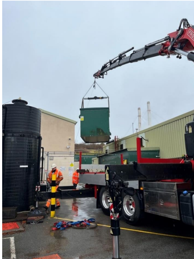
Figure 32 Jekko SPX532 moving the enclosure
