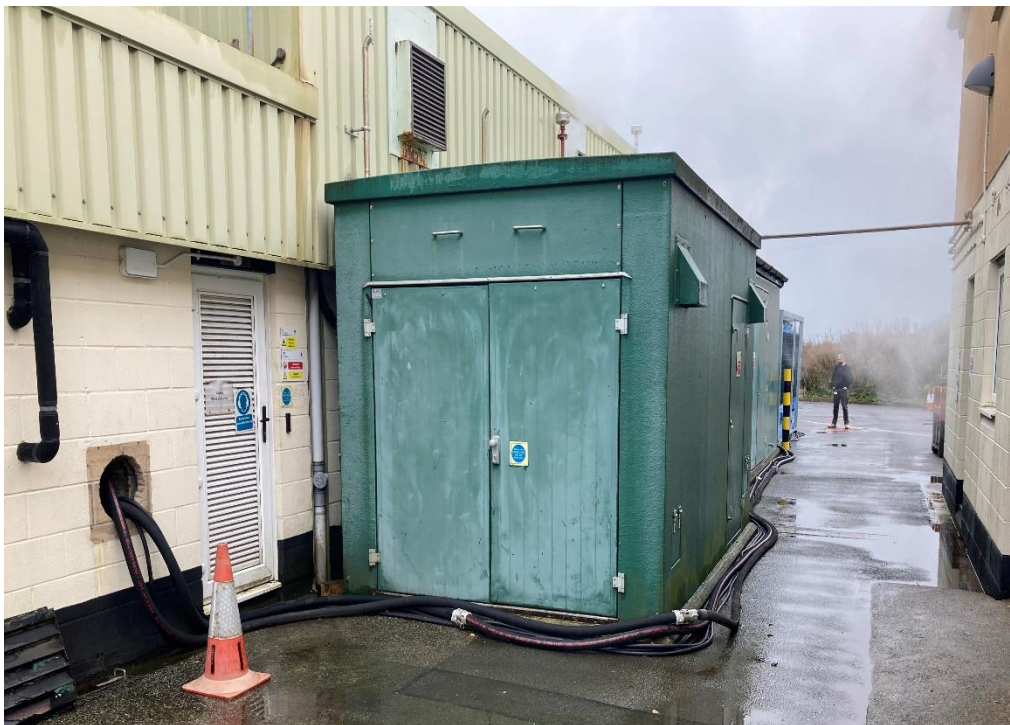
Figure 21 Existing enclosure and Emergency door into plant room
