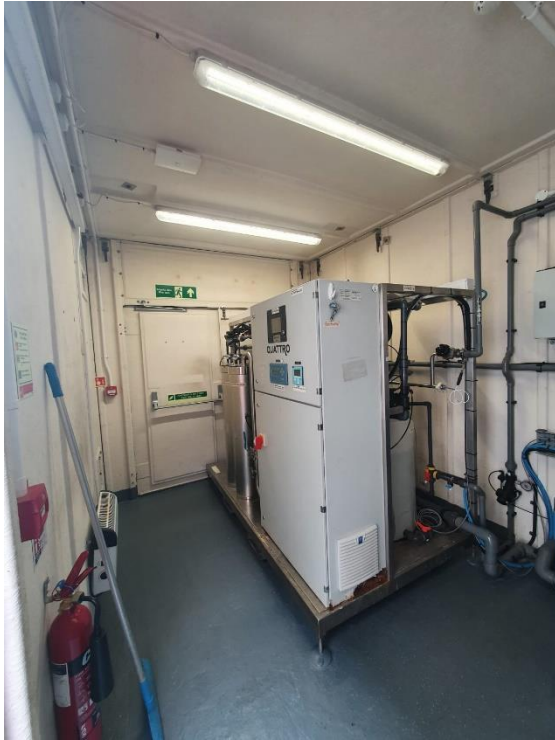
Figure 26 Quattro in place before removing - angle A
