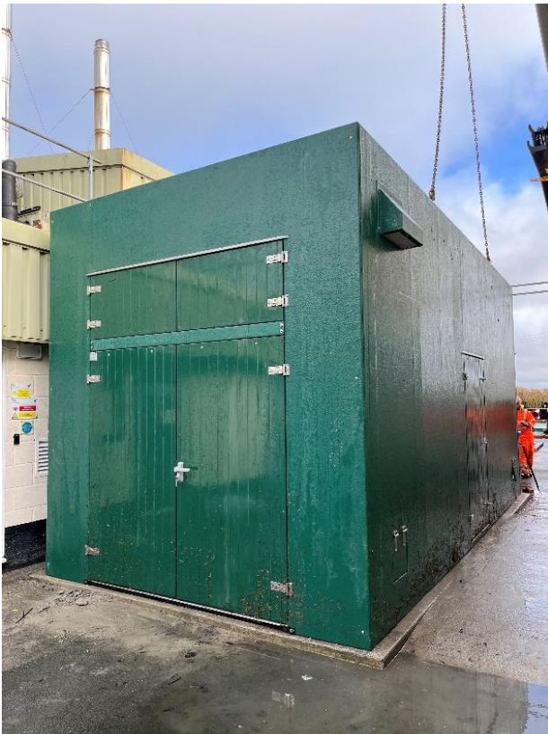
Figure 35 The larger glass reinforced plastic enclosure in place to accommodate the Orion
