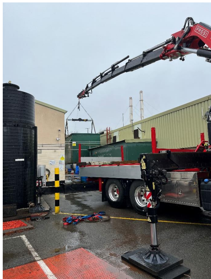
Figure 30 Jekko SPX532 lifting the enclosure
