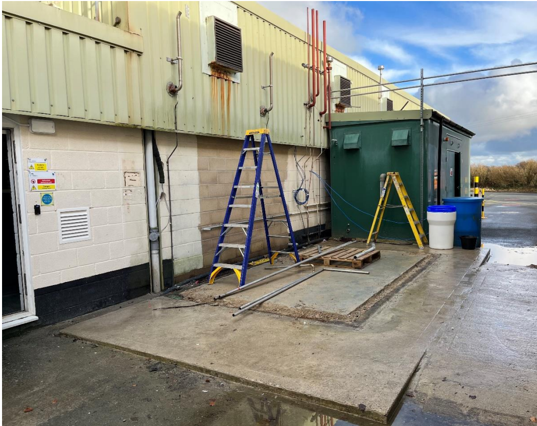
Figure 34 All utilities and glass reinforced enclosure removed
