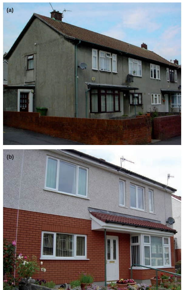
Figure 1: Woolaway houses, Caerphilly: (a) before and (b) after refurbishment
