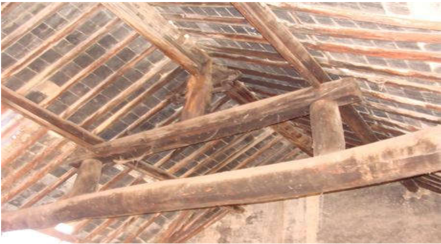
Fig. 1. The beams and rafters of the front hall.
