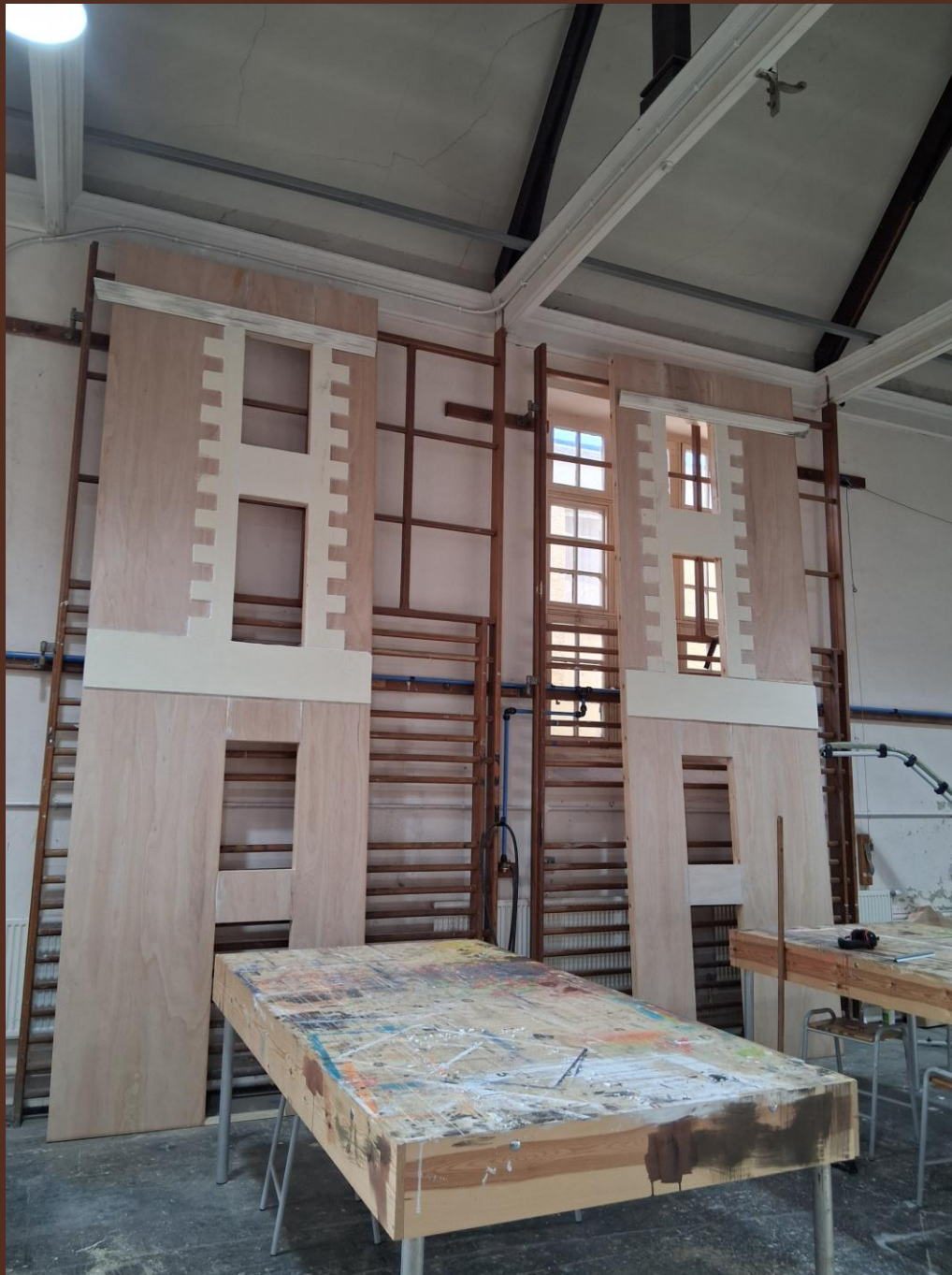
Finished side flats
