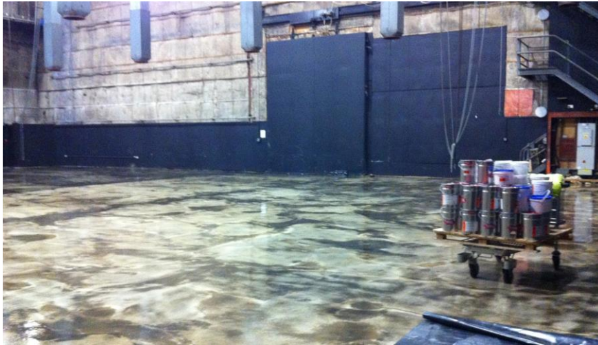
Laser-levellled resin flooring in Stage 9
