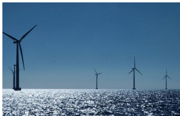
Wind turbines off Denmark. PHOTO: TOM LITTLE/REUTERS
