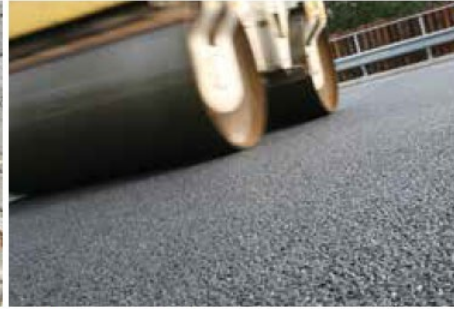
b Porous asphalt
