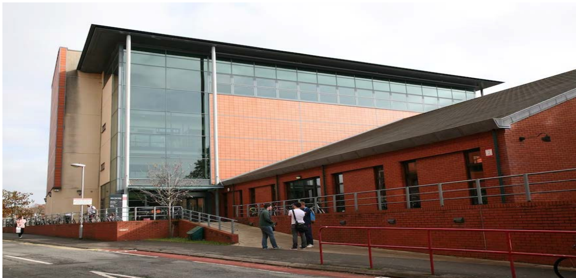
Julian Hodge Building Illustrating the Old and New Sections of the Building / Asset.
