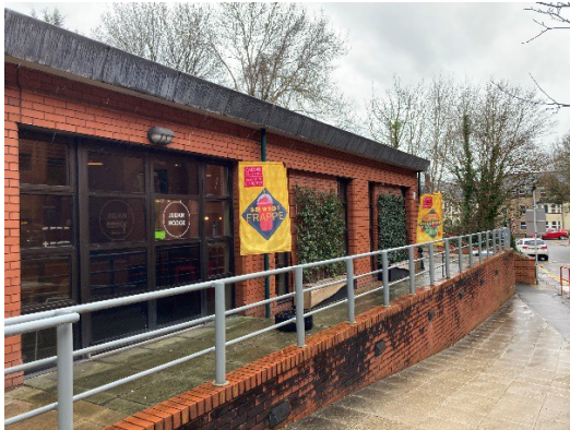
Front Area of the Building
