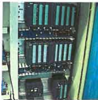
Fig.3 Example of Rack-Mounted PLC- http://www.oocities.org/~buttonbill/m110b.htm
