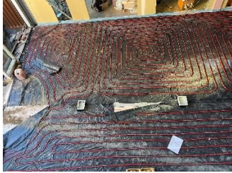
Figure 12 Underfloor heating.
