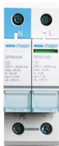
Figure 4- Surge Protection Device (Hager UK, 2024)
