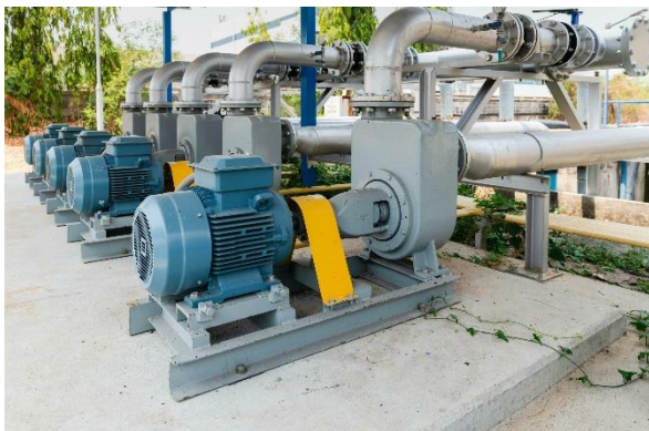
Figure 12:Wastewater pump
