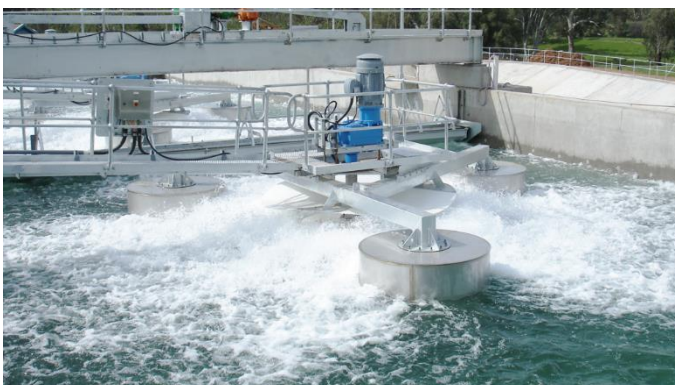
Figure 13:Surface aerator
