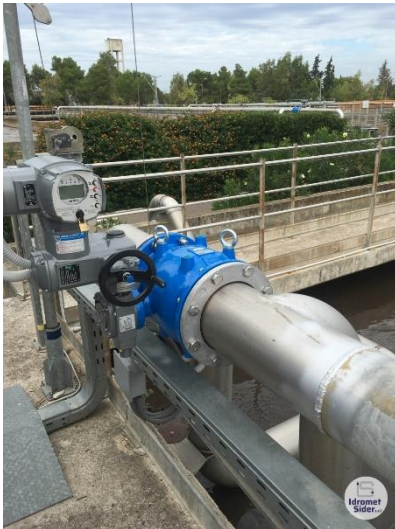
Figure 11:Control valve
