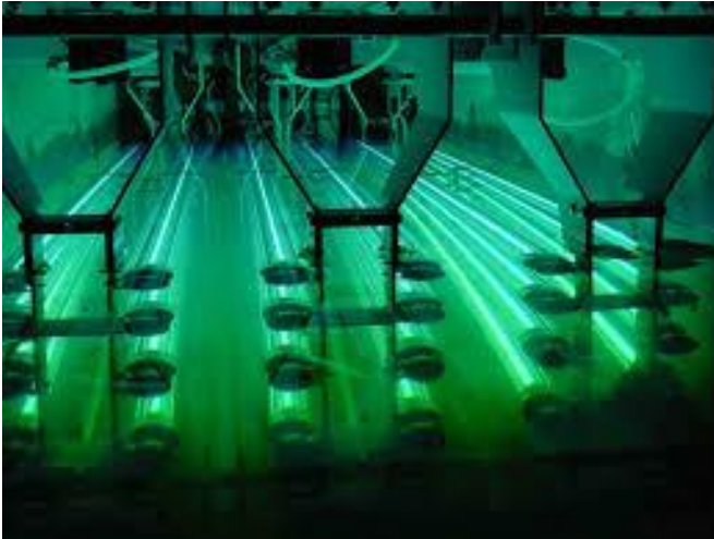
Figure 14:UV Disinfection system
