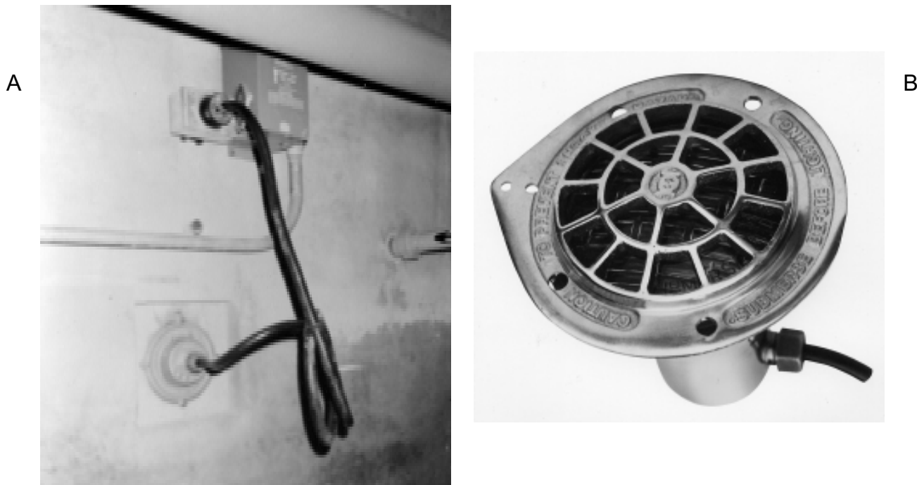
Fig. 3-14. A, Dry niche underwater lighting fixture. B, Wet niche underwater lighting fixture. (Photo courtesy of KDI Paragon, Pleasantville, NY.)
