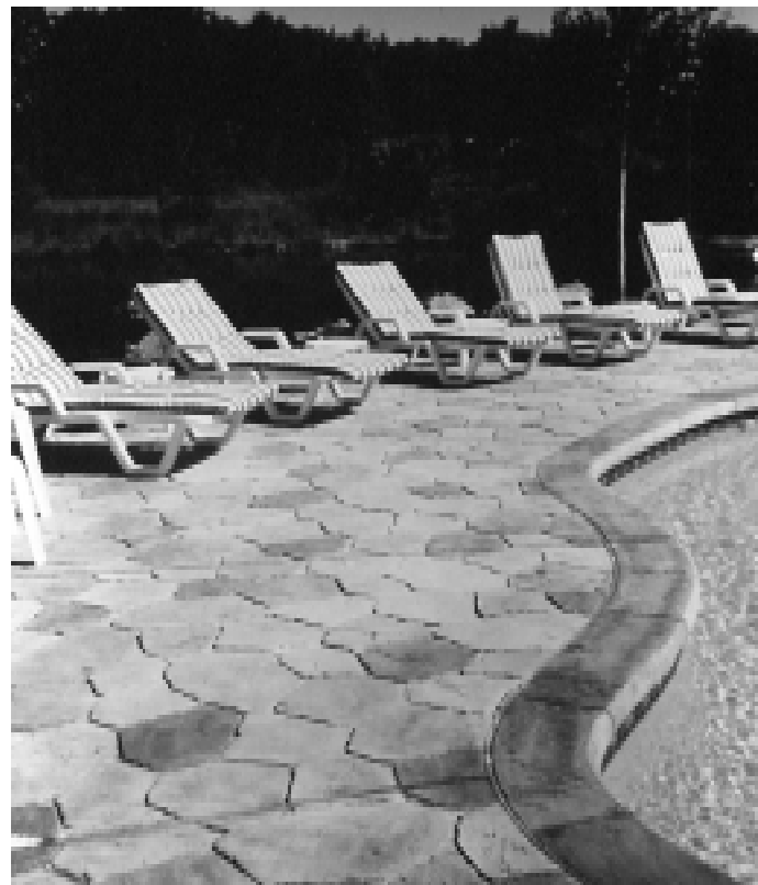
Fig. 3-12. Coping divides the deck from the pool. (Photo courtesy of Bomanite, Madera, Calif.)
