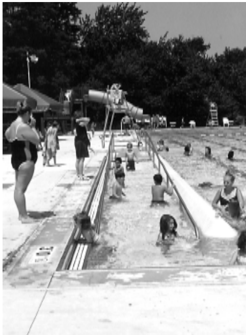
Fig. 3-1. A, Access ramp may be needed to comply with the ADA. B, Chair lifts may be used when pool space is at a premium. (A, Photo courtesy of Water Technology, Inc.; B, photo courtesy of Arjo, Morton Grove, Ill.)
