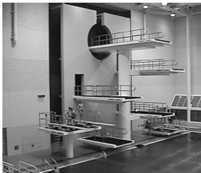
Fig. 3-7. Separate diving well with competitive spring boards and towers at the University of Georgia. (Photo Courtesy of Counsilman & Hunsaker)
