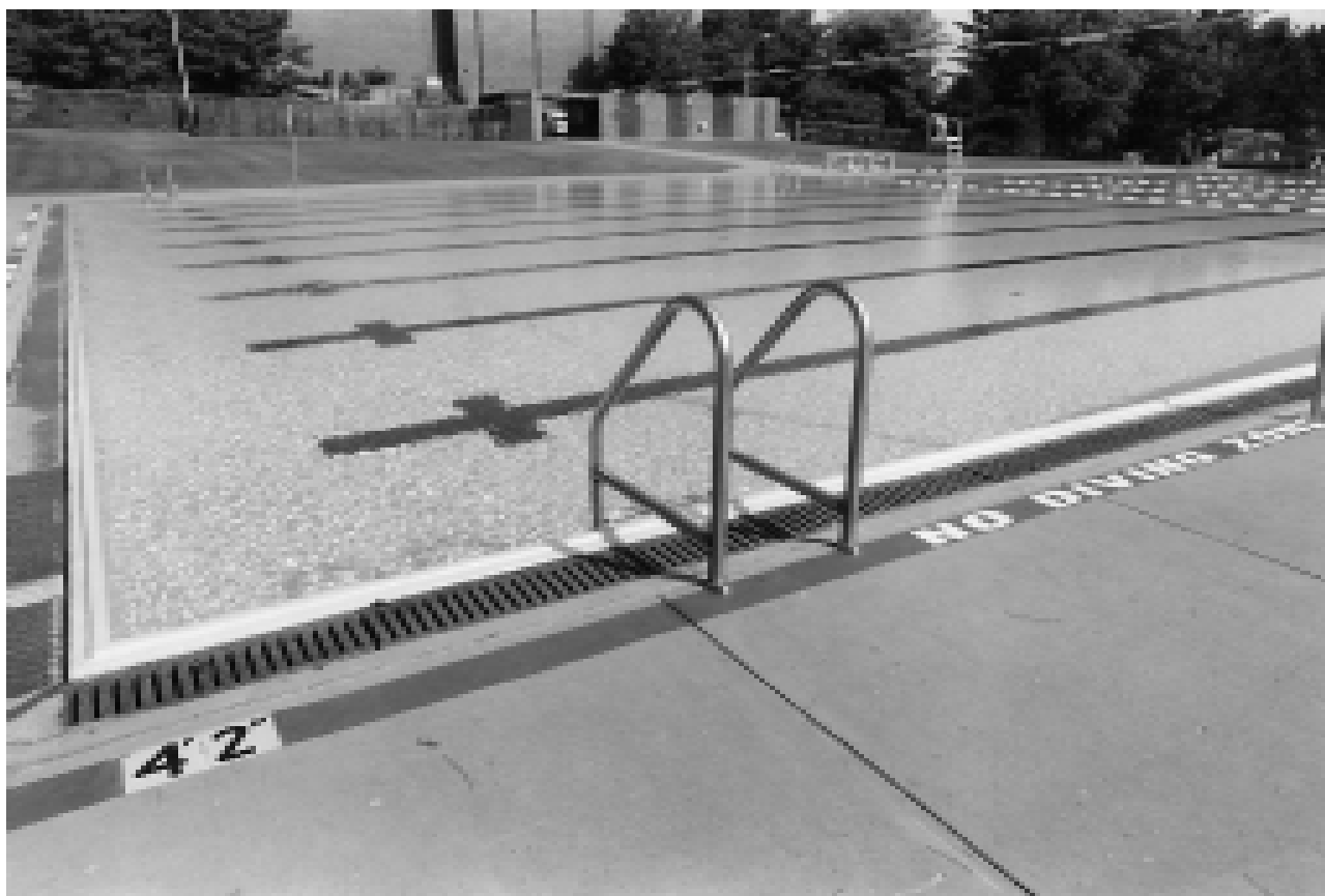
Fig. 3-15. Depth markers and no diving zone painted on pool deck.
