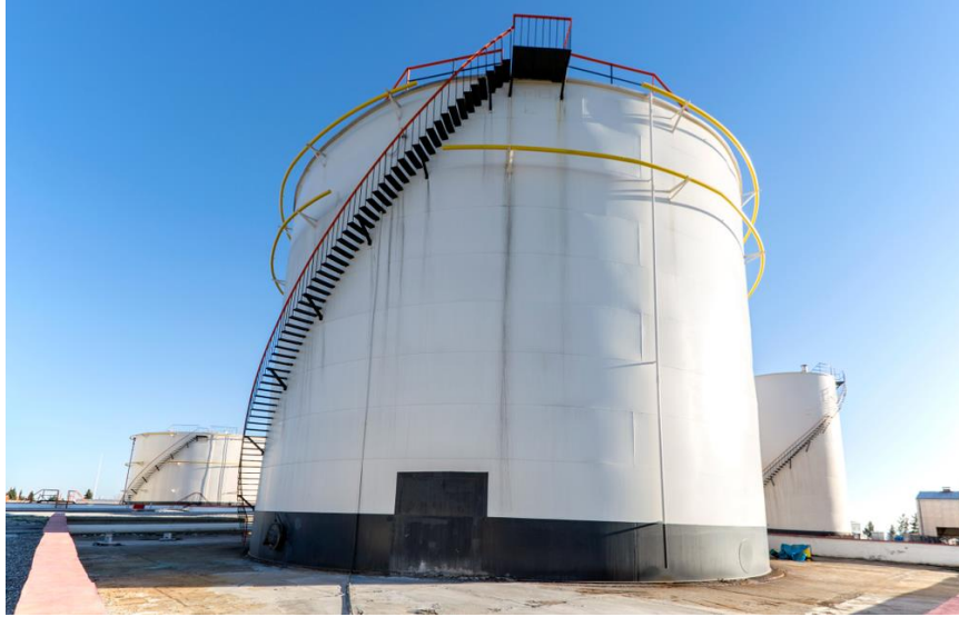
Figure 3: Above Ground Storage Tank [7]
