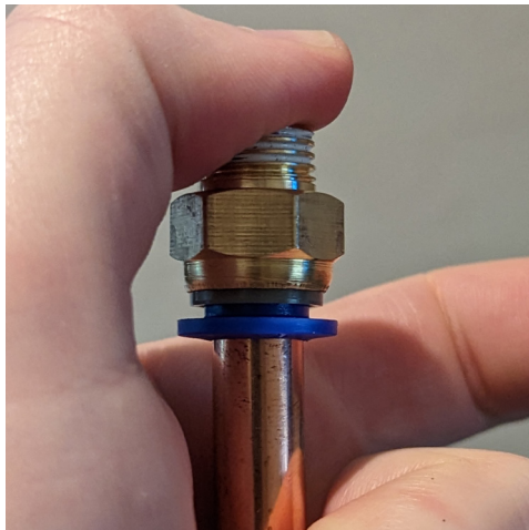
Before pushing onto copper pipe.
