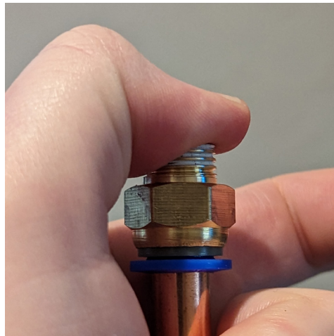
After pushing onto copper pipe. - Note blue plastic is pushed to brass fitting.
