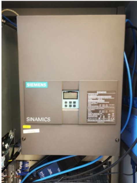
Appendix Figure 17 - Siemens 3-PH DCM Drive
