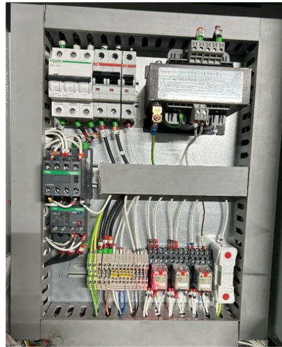
Figure 16 - Completed System Wiring
