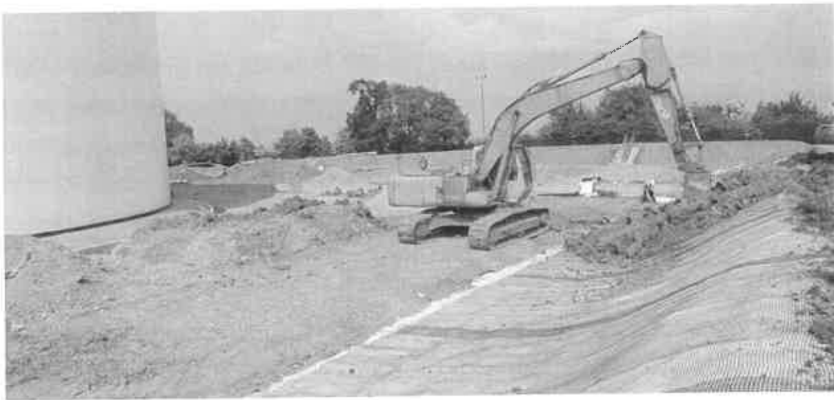
Impermeable layer being installed in a tank bund.
