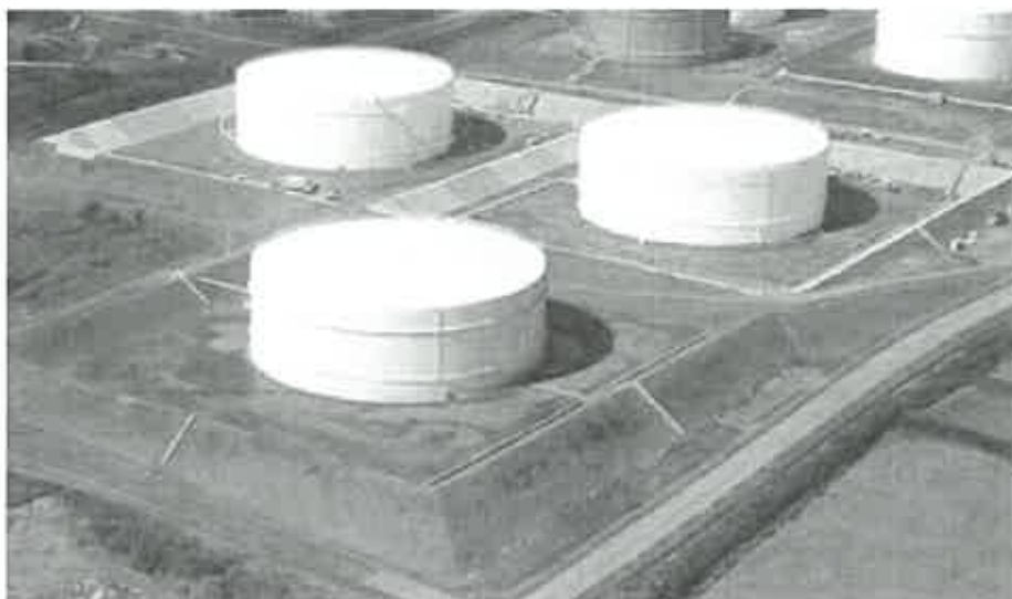
Tanks in bunded areas at Valero Pembrookshire Oil Terminal (VPOT)
