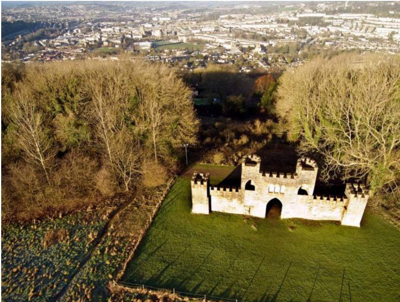
Sham Castle, Bath, by Ralph Allen, 1762: aerial view
