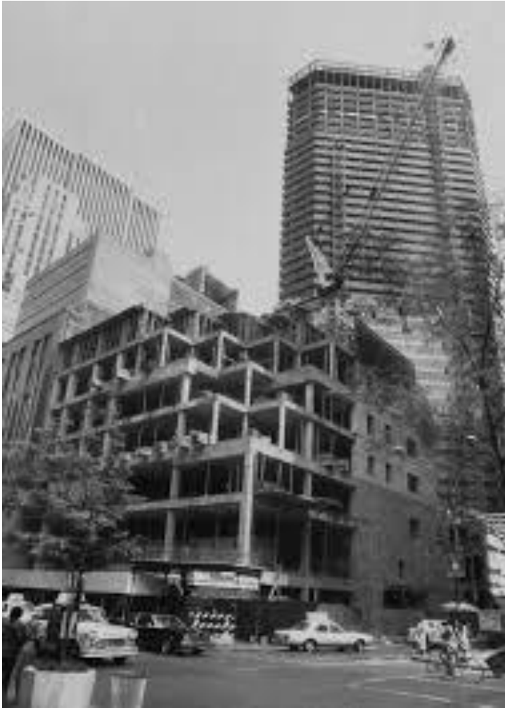
Trump Tower, New York City by Der Scutt of Poor, Swanke, Hayden & Connell, 1983: construction
