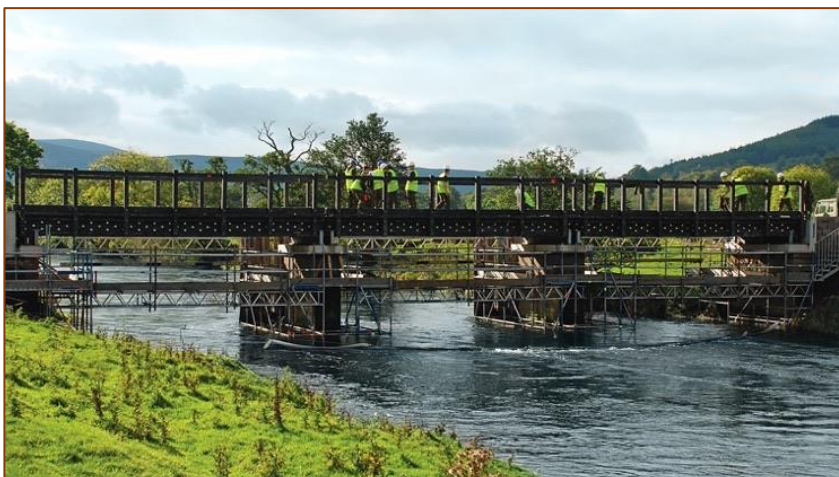
Figure 20 The Easter Dawyck Bridge, the longest in the world built using recycled plastic. Photo: Sicut / Veritech LTD.
