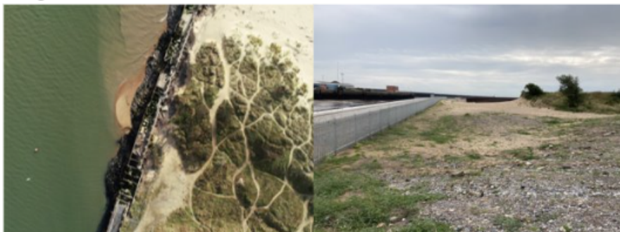
Aerial image of site before construction by Richard Youle
