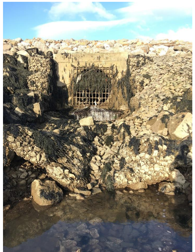
Figure 34-Penstock emptying into bay (Low tide)
