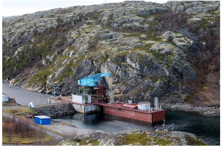
Figure 15-Kislaya Guba Tidal Power Plant. (Unknown, 2019)
