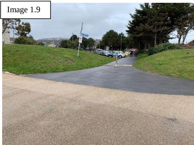
Image 1.9: Cycle/footway between both car parks
