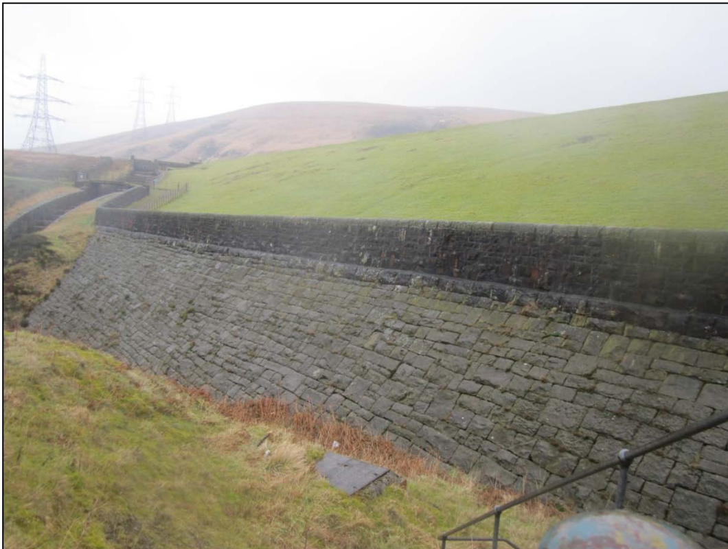
Plate 6: Detail of Gorpley Reservoir dam (Site 43).
