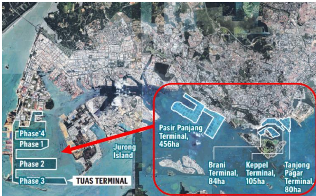
Figure 30: Overview of the Tuas Terminal
