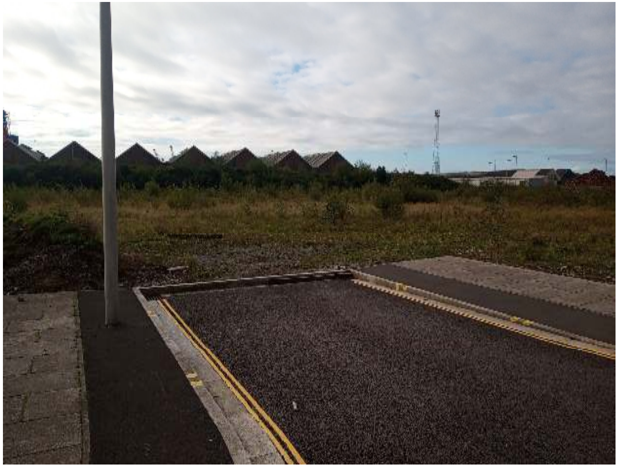
(Site photograph 2, Cullen, 2021)
