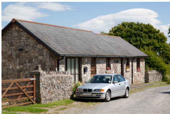
Below: Stone walls providing enclosure for private space, converted barn Oxwich Green
