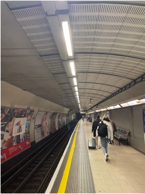
Figure 2a. Kings Cross St Pancras eastbound platform
