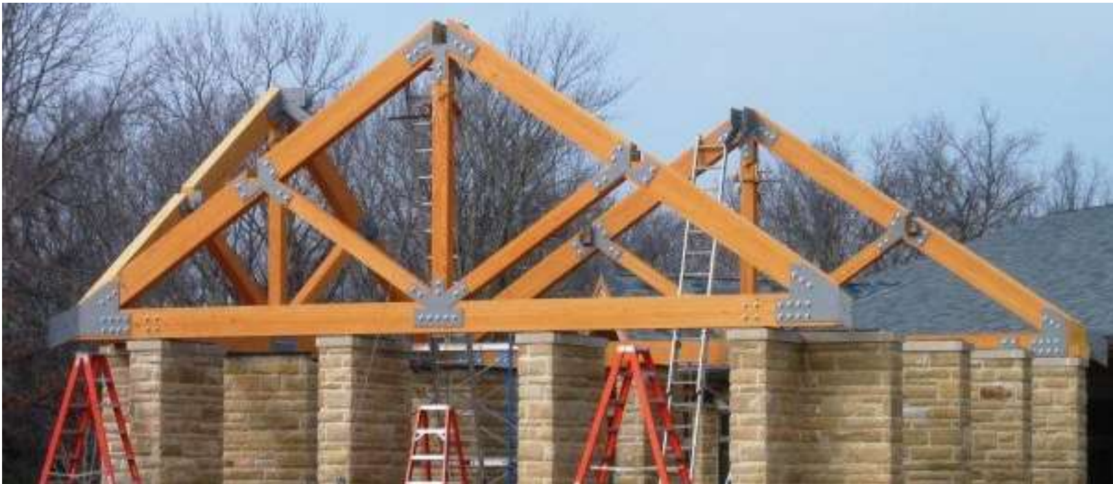
King Post Truss
