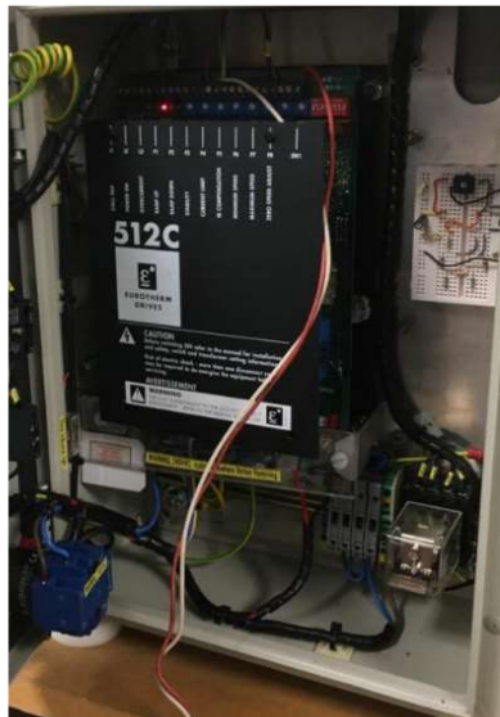
Figure 27 - Practical investigation into a Single quadrant DC Drive - Parker 512C
